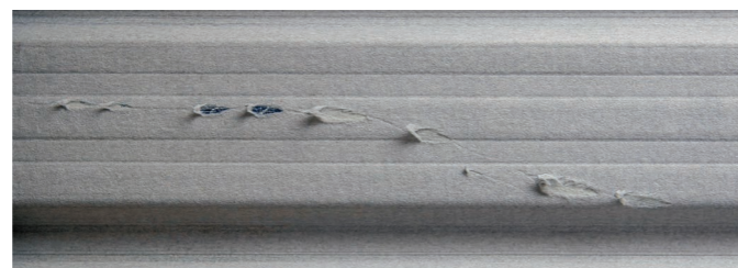
An example of minor damage that can be fixed
